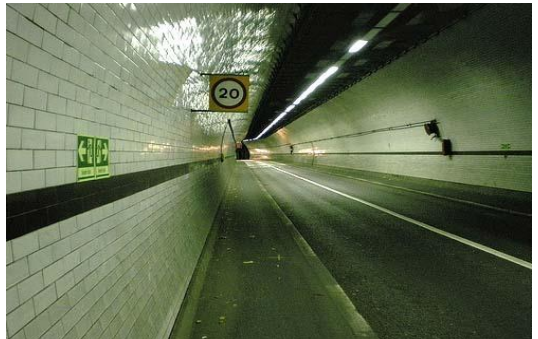
Rotherhithe Tunnel (Fire / Ventilation system renewal) Daily users – 30,000
