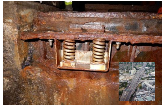
A40 Westway (12 x key bridge Joint renewals) Daily users – 90,000
