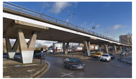
Croydon Flyover (significant structural lighting renewal) Daily users – 40,000
